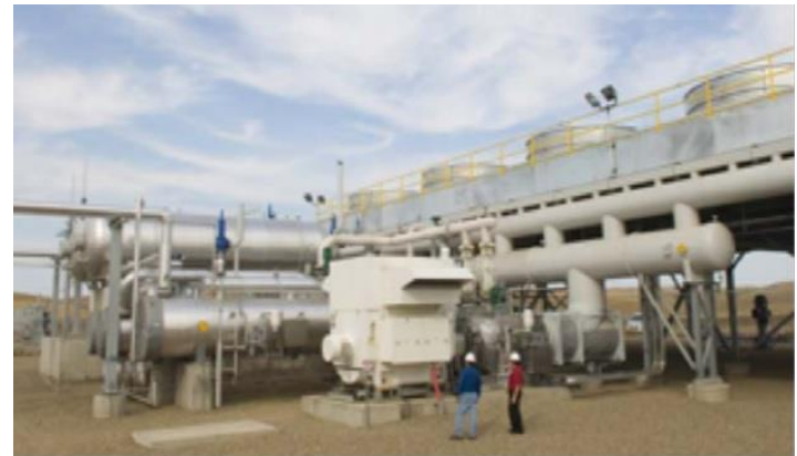
Northern Boarder Pipeline, North Dakota
