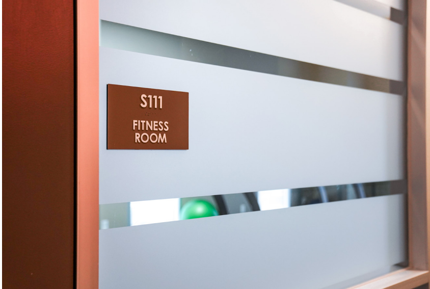
Frosting a portion of glass on the fitness room in Cougar Village 1, Cougar Village 2, Cougar Place, and Moody Towers to address the concerns of our Residential Hall Association (RHA).
