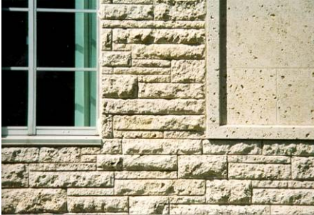
Detail of materials in dormitory group
