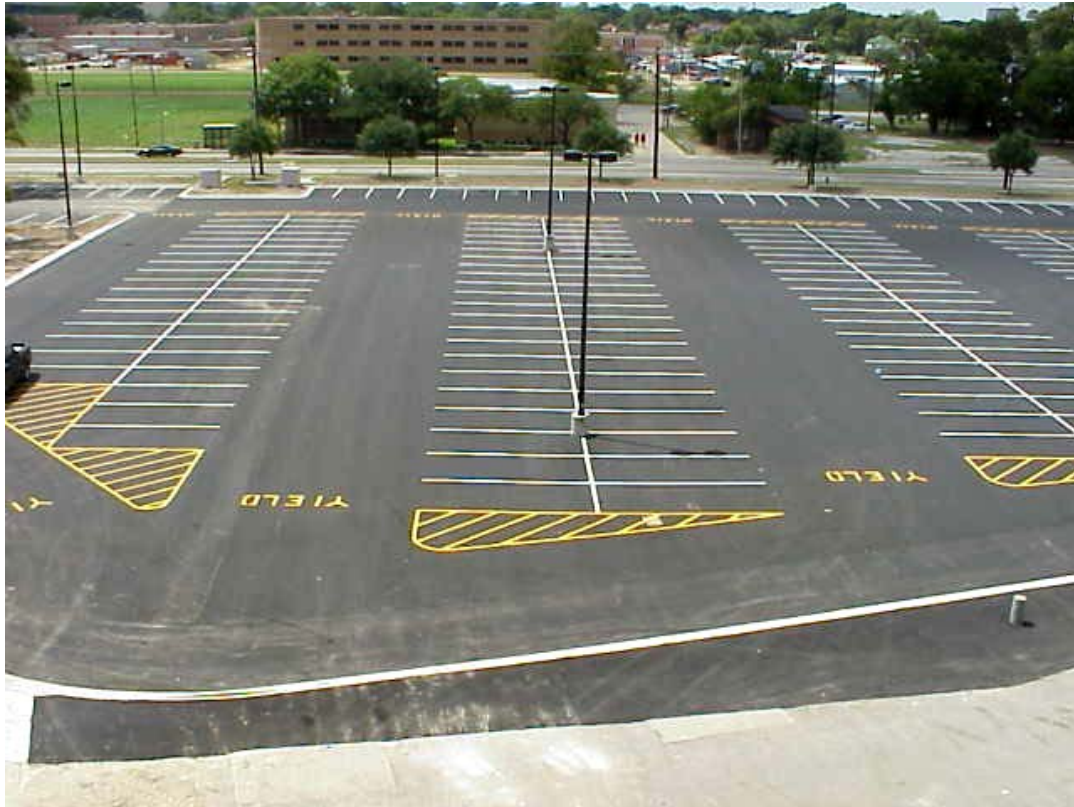
FIGURE 1.1 OVERVIEW OF PARKING LOT AND LIGHTING
