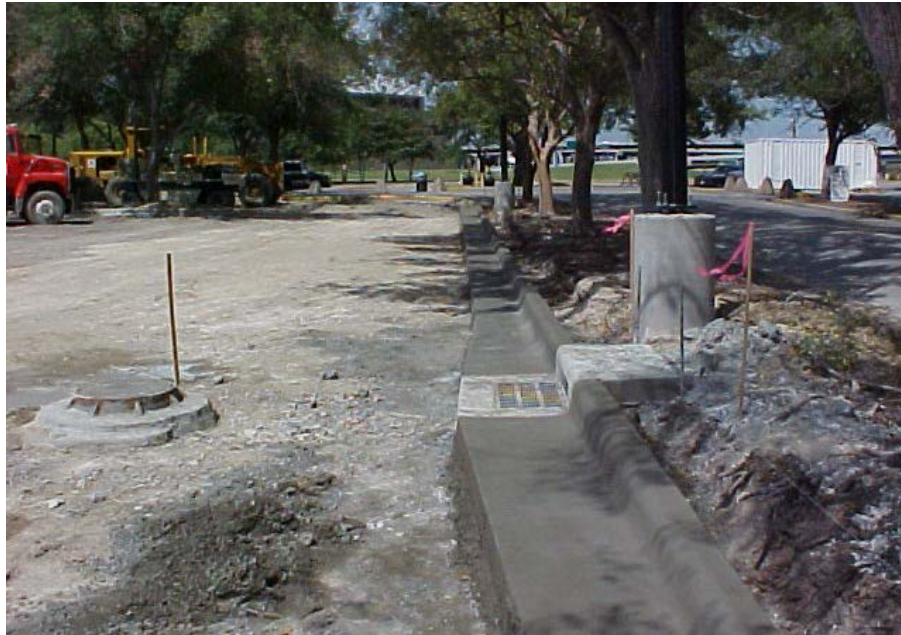
FIGURE 9.8.2 MONOLITHIC CURB, INLET AND CATCH BASIN
