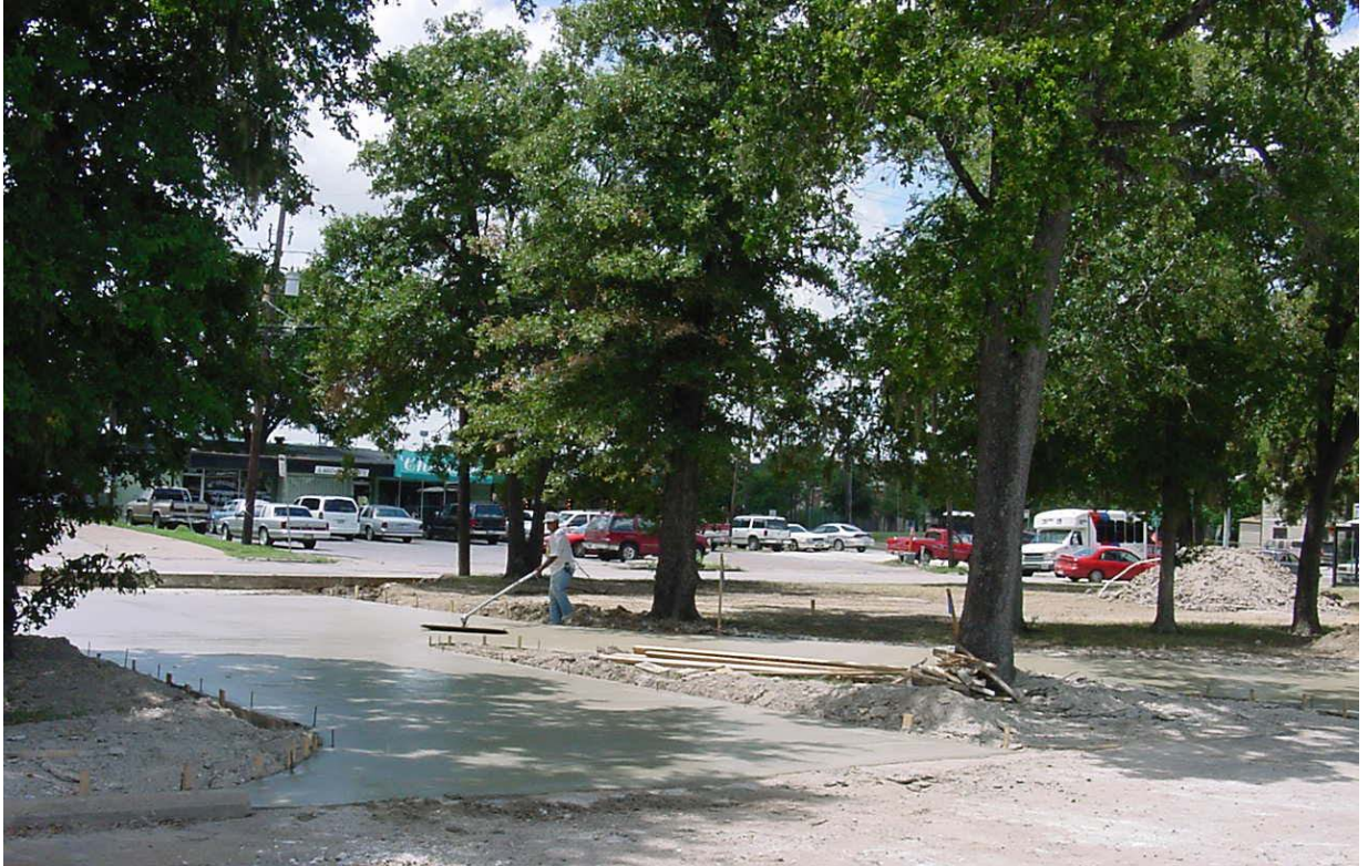
FIGURE 9.2.2 FINISHING CONCRETE AT WHEELER STREET DRIVEWAY
