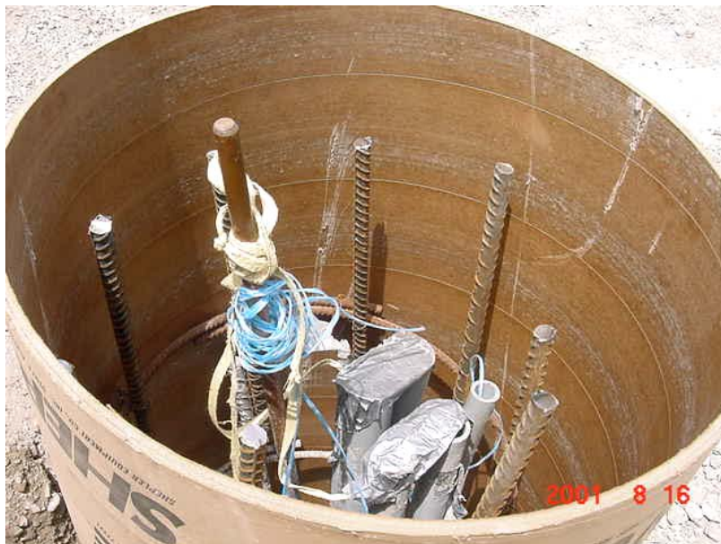
FIGURE 9.9.4 REBAR, ELECTRICAL CONDUIT
