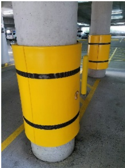
FIGURE 9.2.9 CONCRETE-FILLED BOLLARD
