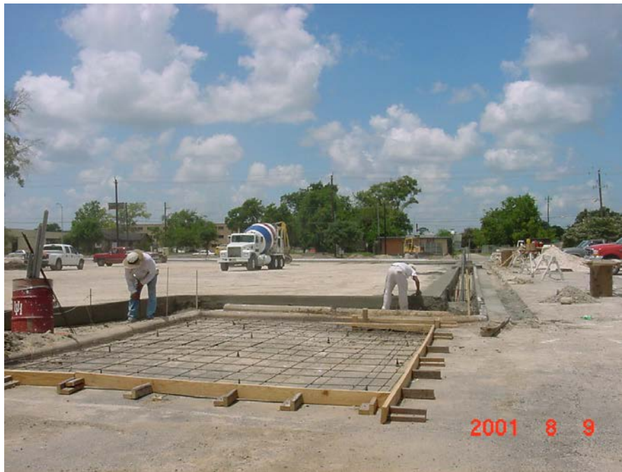
FIGURE 9.6.1 FRAMING AND REINFORCING FOR CONCRETE PAD
