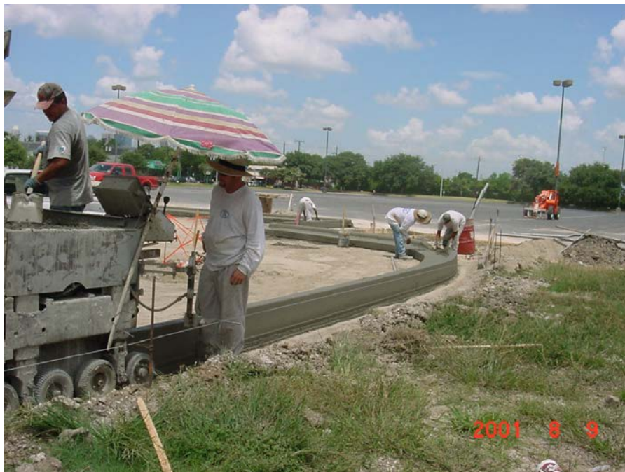
FIGURE 9.2.8 MONOLITHIC CURB ALONG PERIMETER OF PARKING LOT
