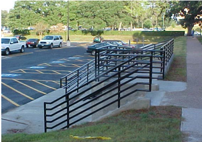
FIGURE 9.3.1 SHARED HANDICAPPED ACCESS AISLES LEADING TO RAMP
