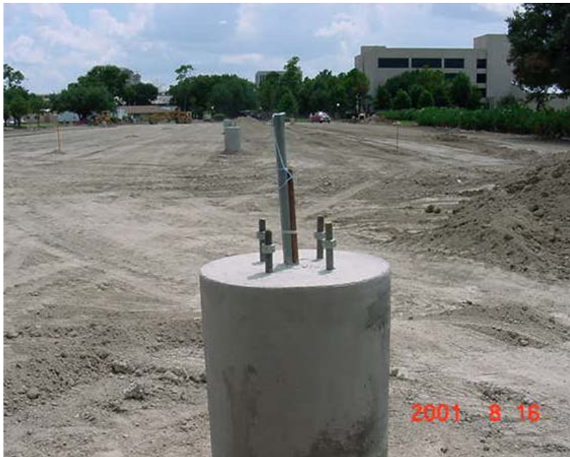
FIGURE 9.9.5 CONCRETE LIGHT POLE BASE WITH ANCHOR BOLTS
