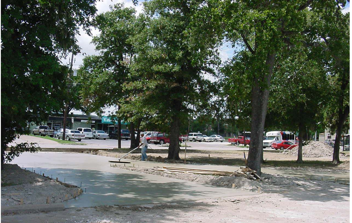
FIGURE 9.2.2 FINISHING CONCRETE AT WHEELER STREET DRIVEWAY
