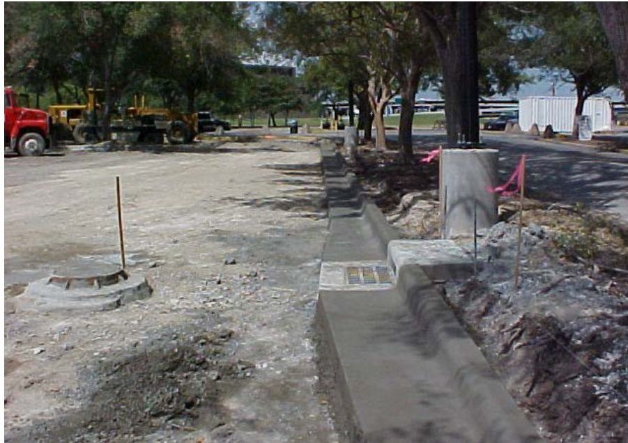
FIGURE 9.8.2 MONOLITHIC CURB, INLET AND CATCH BASIN
