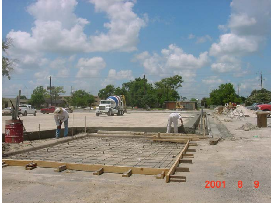
FIGURE 9.6.1 FRAMING AND REINFORCING FOR CONCRETE PAD
