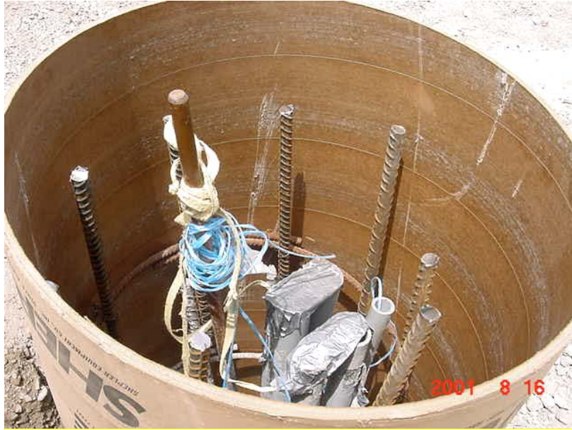
FIGURE 9.9.4 REBAR, ELECTRICAL CONDUIT
