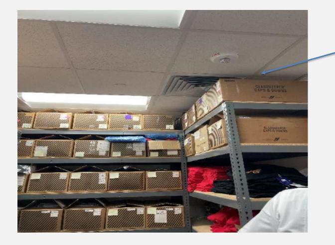
Storage stacked too high. There should be 18 inch clearance from sprinkler heads.
