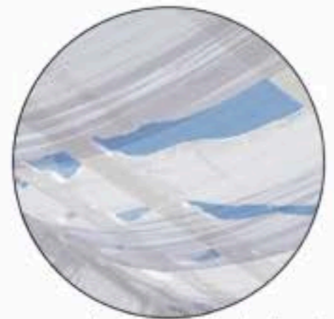
Drapes used as adjustable shading in a third roof condition.
