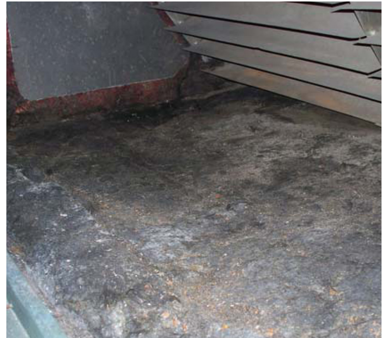
Fraying ductliner
