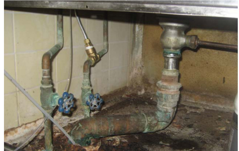
P2: Drains below sinks
