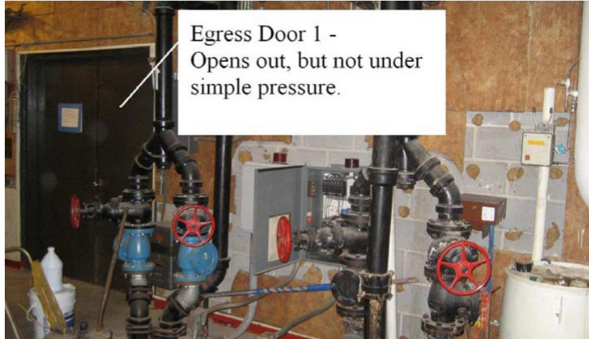
E7: Egress path 1 from Main Electrical/Mechanical Room.
