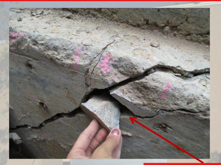
Another View of Failed Grade Beam Measured to have a 4 inch slope
