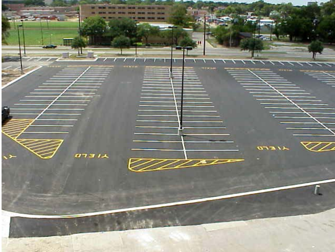
FIGURE 1.1 OVERVIEW OF PARKING LOT AND LIGHTING
