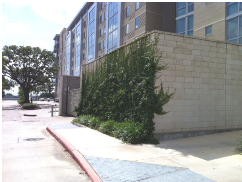
FIGURE 6.7.6 SERVICE AREA SCREENING
