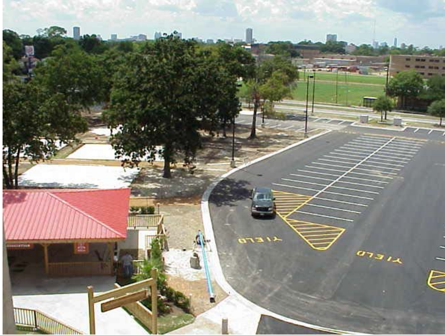
FIGURE 9.10.2 YIELD MARKINGS AND YELLOW STRIPING
