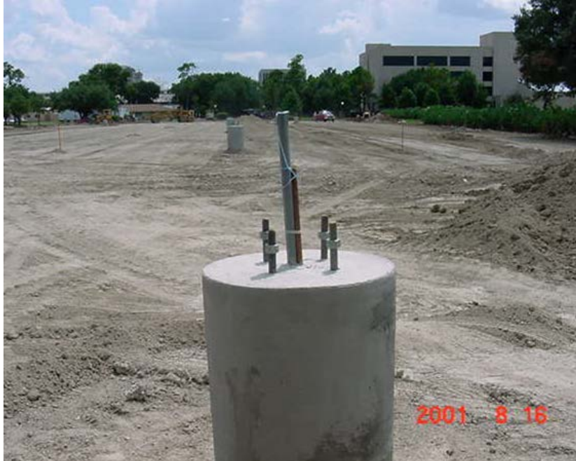
FIGURE 9.9.5 CONCRETE LIGHT POLE BASE WITH ANCHOR BOLTS
