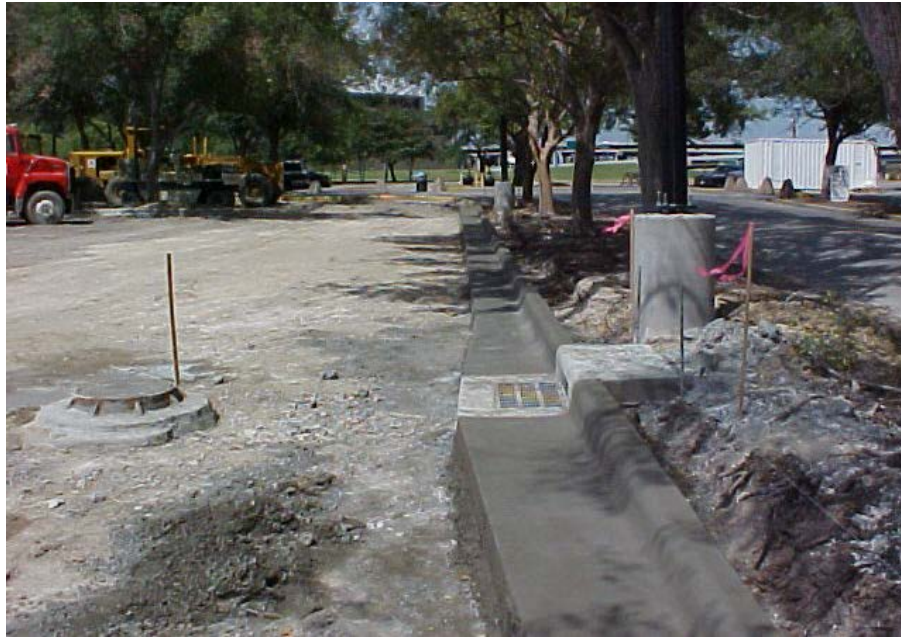
FIGURE 9.8.2 MONOLITHIC CURB, INLET AND CATCH BASIN
